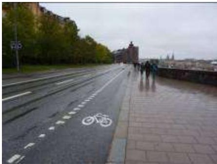
This main stretch has wide segregated cycle lanes on both sides flowing with the traffic. Interestingly the near side lane was within the road boundary but the far was on the pavement. This shows a sensible flexible design approach to maximise space.
