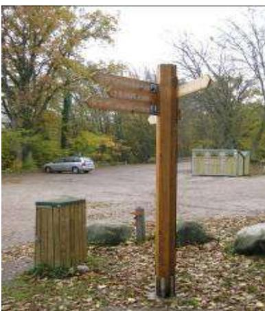
A prototype fingerpost in Stenshuvud NP. This shows the hexagonal pillar design EPA are considering as a standard.
