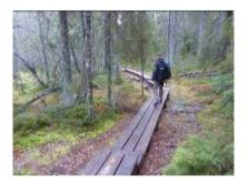
Boardwalk was used by all locations visited in Sweden and here in Tyresta we can see a typical three plank width construction with steps.
