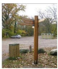
A prototype fingerpost in Stenshuvud NP. This shows the hexagonal pillar design EPA are considering as a standard.
